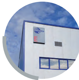
A new autonomous storage building of 4,500 m 2
